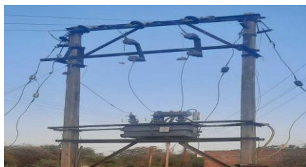
Fig.18 RCC Double Pole Distribution
